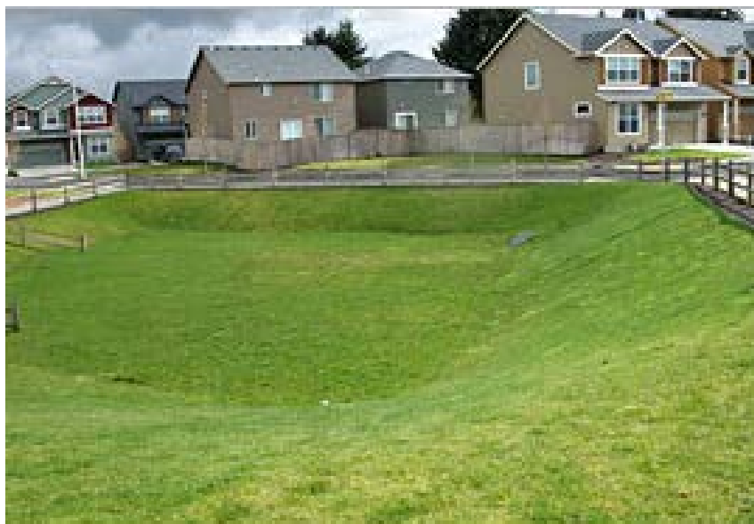
Figure 4: Example of a Dry Detention Pond ("Detention Pond")
