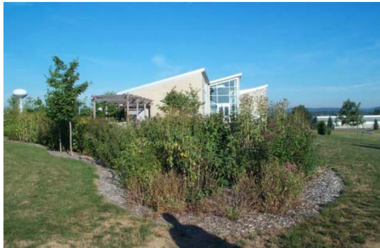
Figure 3: Example of a Large Rain Garden ("Pennsylvania Stormwater Best Management Practices Manual")
