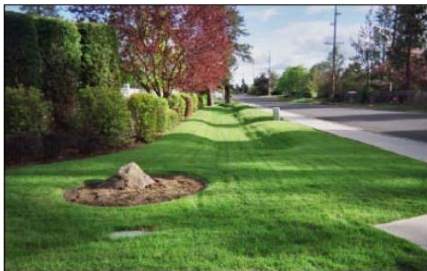
Figure 2: Example of a Grass swale "Reducing Stormwater Runoff and Pollution through Low Impact Development."
